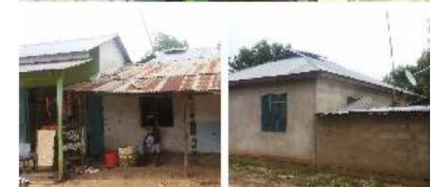
User who improved his mud walled house to brick structure
